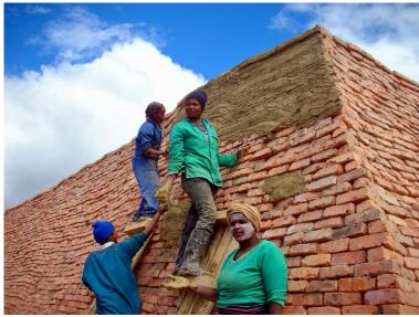
It takes about 3 weeks to build a Clamp Kiln with a load of up to 450,000 bricks. Larger loads tend to used in the summer as dry green bricks are more regularly available. Up to 80% of output is concentrated in the summer months.
