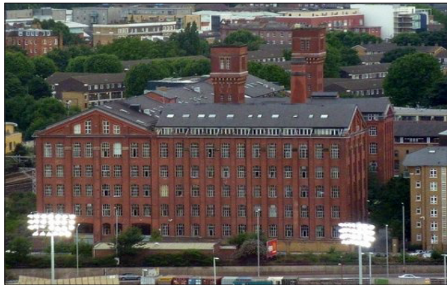
The former Bryant & May factory in Bow as viewed from the Orbit, with the tops of the Olympic Stadium floodlights in the foreground.
