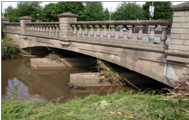
Dogpole Lane Bridge
