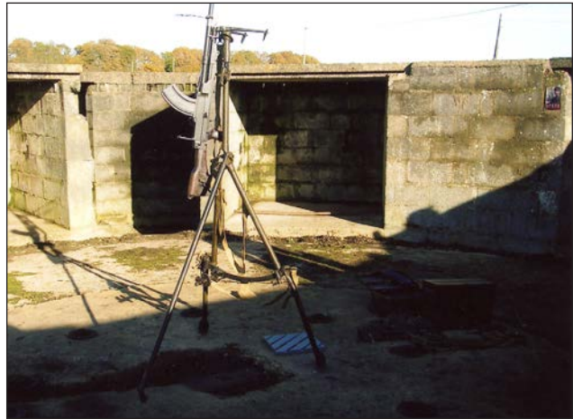
3.7" Emplacement. The receptacles surrounding the concrete plinth were for ammunition storage. At Goodrest Farm there were at least four emplacements, with just possibly a fifth.
