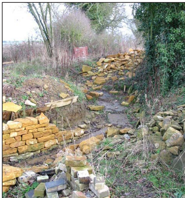
Restoring the exit ramp
