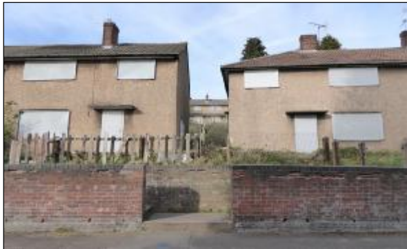
Former miners' housing in Camp Hill, Nuneaton, due for demolition.
