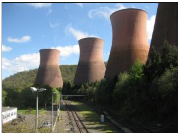
Ironbridge B Cooling Towers on our Visit.
