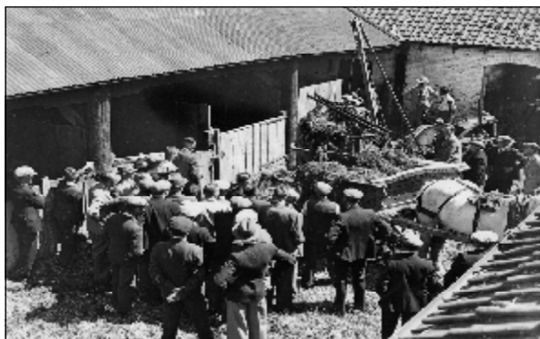
An interested audience for a demonstration of Thwaites lifting machinery.
