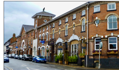
Former Ashwin's warehouse, Union Street.
